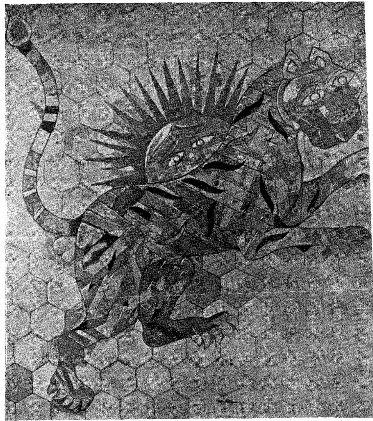
Emblem of Tiger and Rising Sun found on the facade of the Bahamani Throne Palace (Takht-Mahal) at Bidar.
