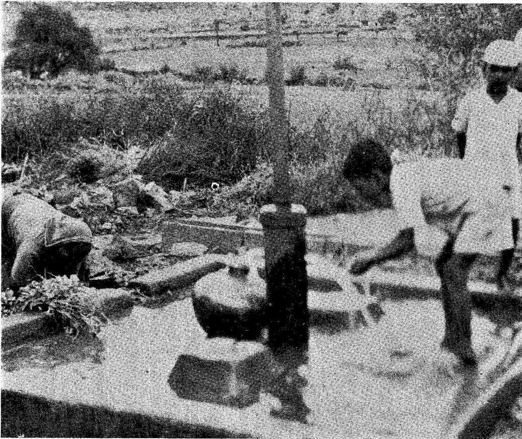
The bore-well at Hallikhed (K) in Humnabad taluk, which is of Artesian condition and is overflowing.
